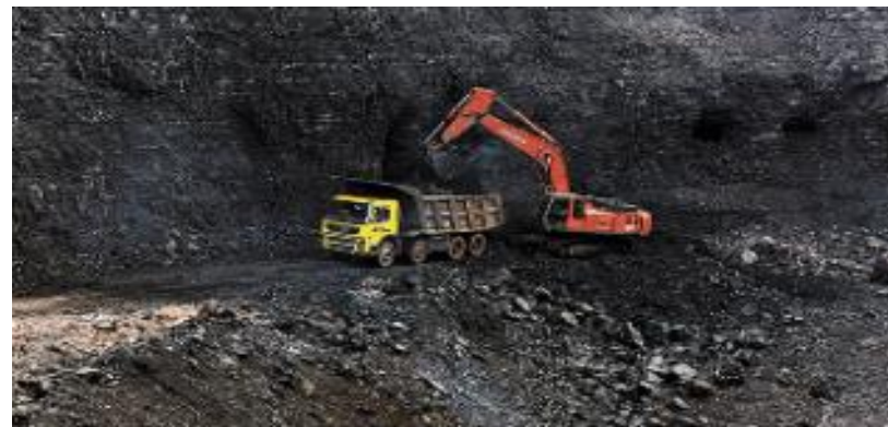
Coal Mines (Total Capacity of 2.04 MMT p.a.)
